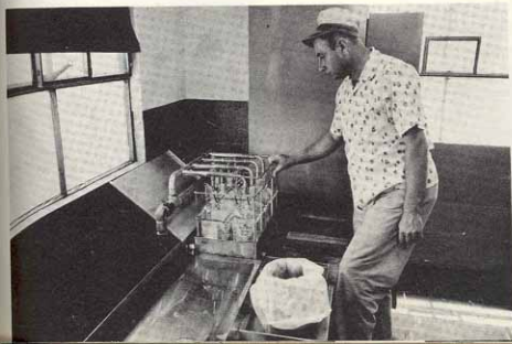
FILLING BOTTLES. Mountain-fresh water flows from spring, through pipes, into bottling plant by force of gravity. It is sent into bottles, 8 at a time, through this multiple spout unit operated by Mr. Hienbaugh. Bottling plant is mile from spring
